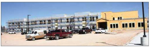
The outside work on the charter school building is progressing. Rigid insulation has been installed on the north end and the stucco base layer has been installed on the eastern and southern side of the buildings. Some of the islands and lighting have been installed in the parking lot.
